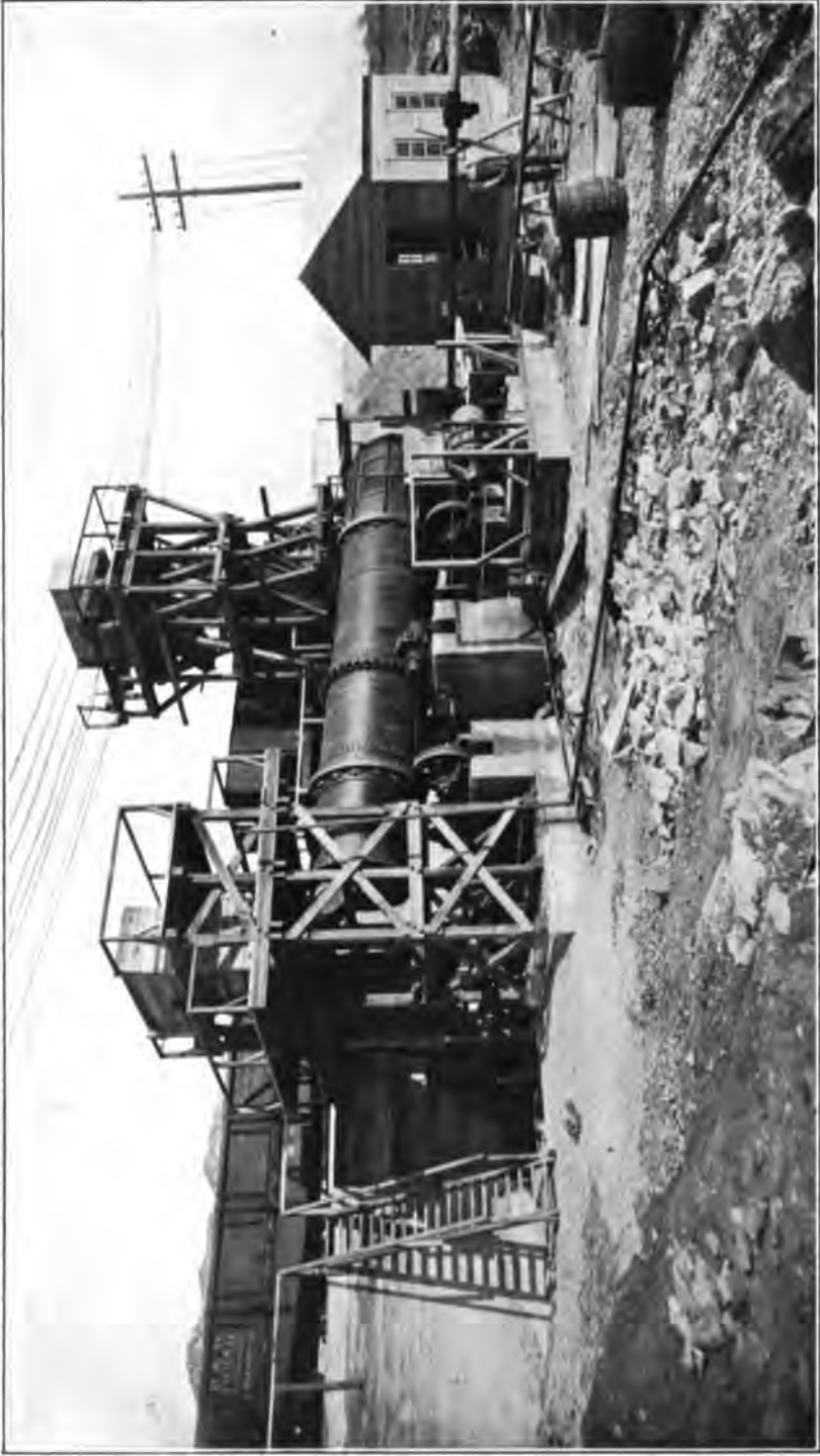
PLATE XXXII.—Washery Plant for Removal of Clay from the Crushed Limestone at National Limestone Company Plant.
